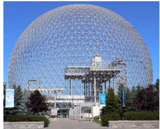
Figure 10.42 Tensegrity structures: (a) a tent; (b) Montreal bio-sphere (Courtesy Mr. Philipp Hienstorfer).
